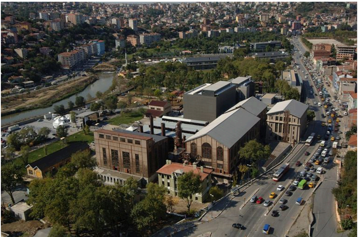
Fig. 24 - The final view of the project
