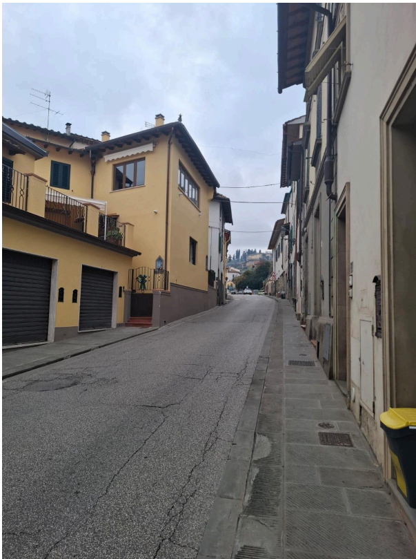
Fig. 17 - Lack of sidewalks
